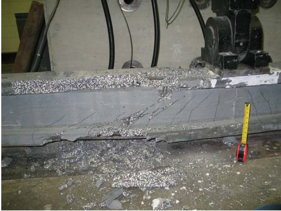
Figure 9. Beam after failure in shear
