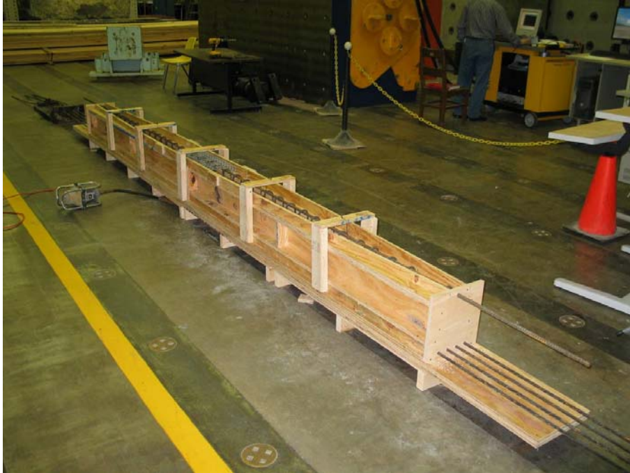
Figure 2. Beam formwork and reinforcement prior to concrete placement
