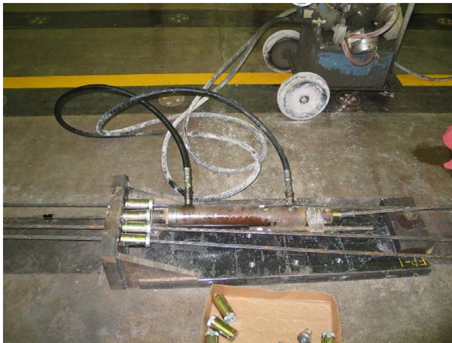
Figure 1. Stressing of reinforcing strands with a hydraulic jack
