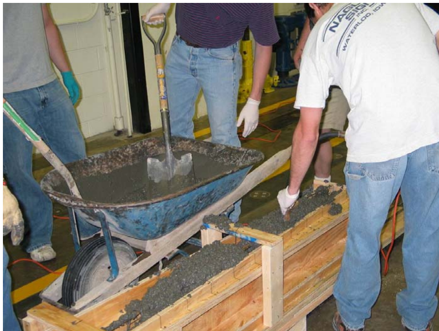
Figure 3. Placement of concrete
